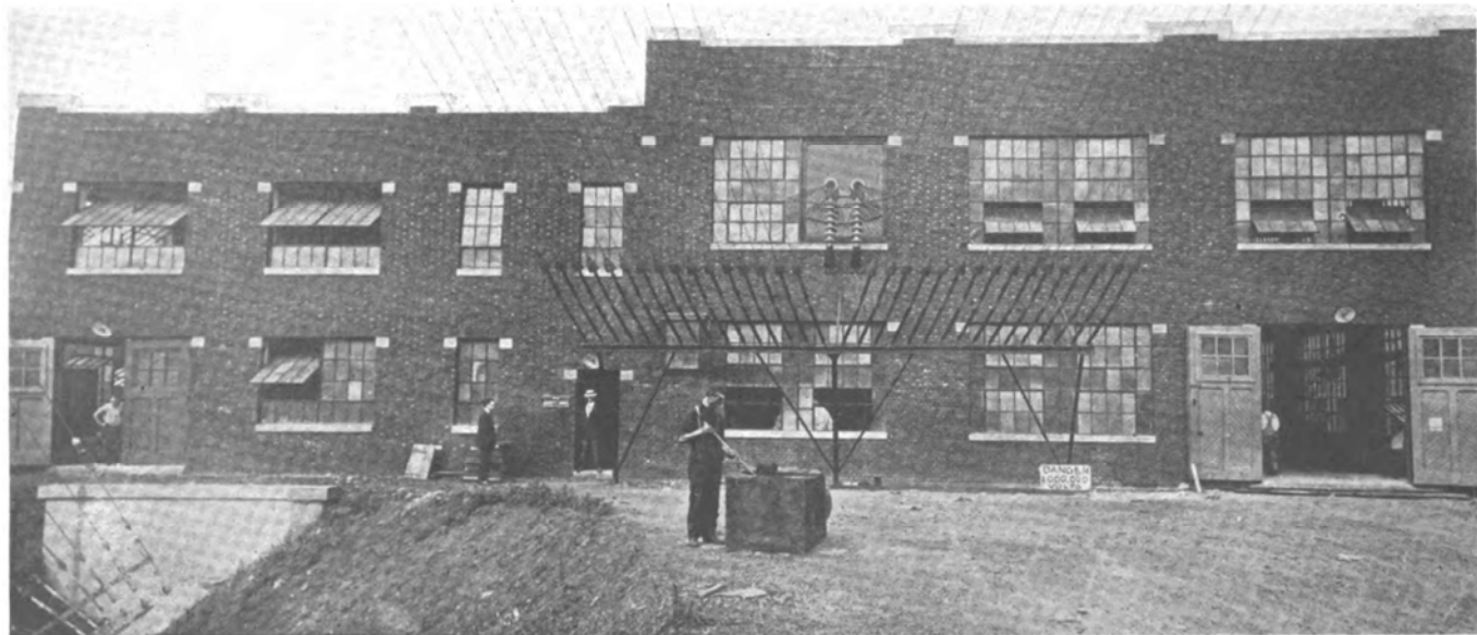
Transmitter Building “The Power House”
