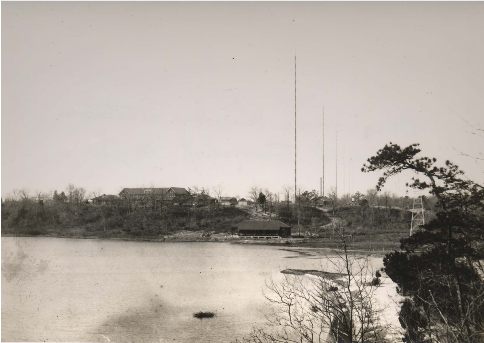
View of the station from the east side of the Shark River, ca. 1914. Operations building is at the water's edge, with mile-long main antenna behind it. One of the lattice work towers for the balancing-out antenna is visible behind the tree to the right. The "hotel," station manager's and chief engineers cottages, and the power plant are on the high ground.
