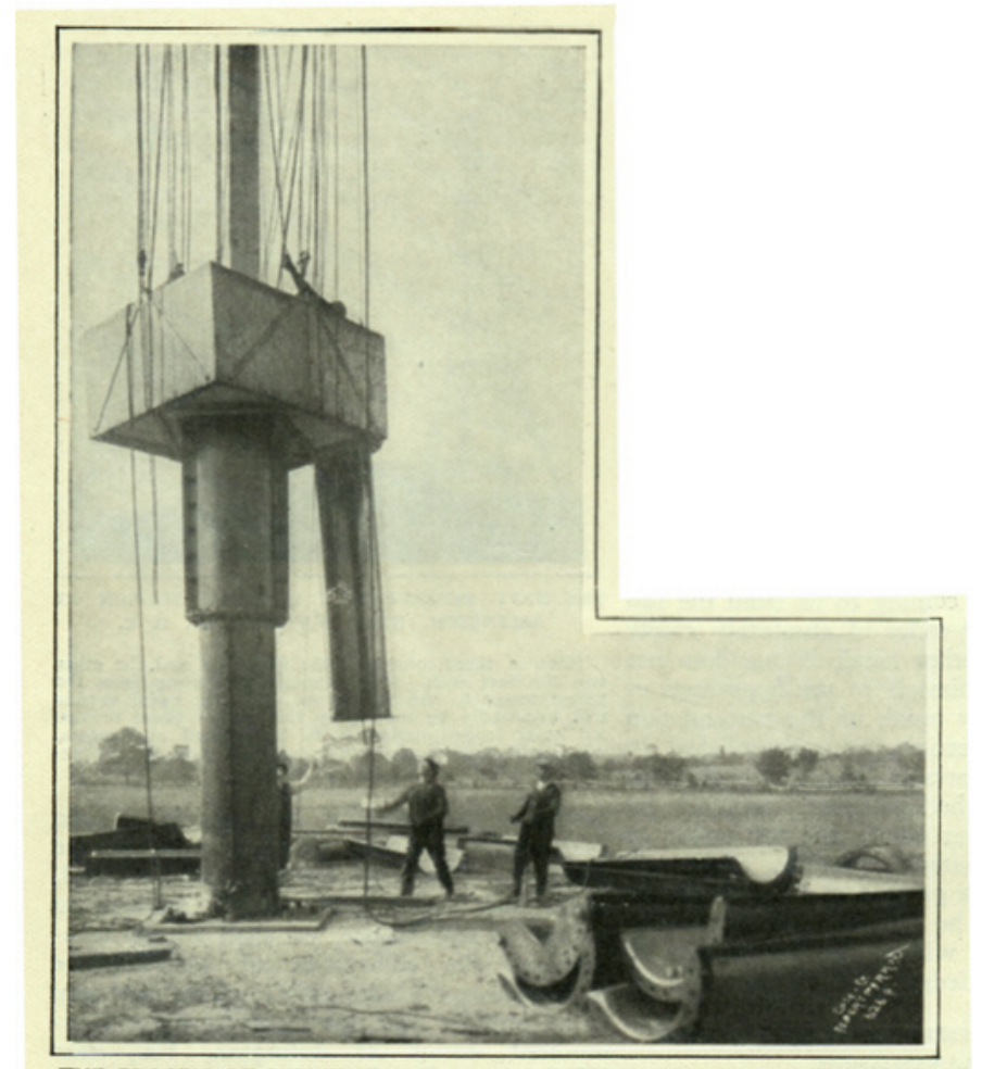
Erecting the steel masts.
