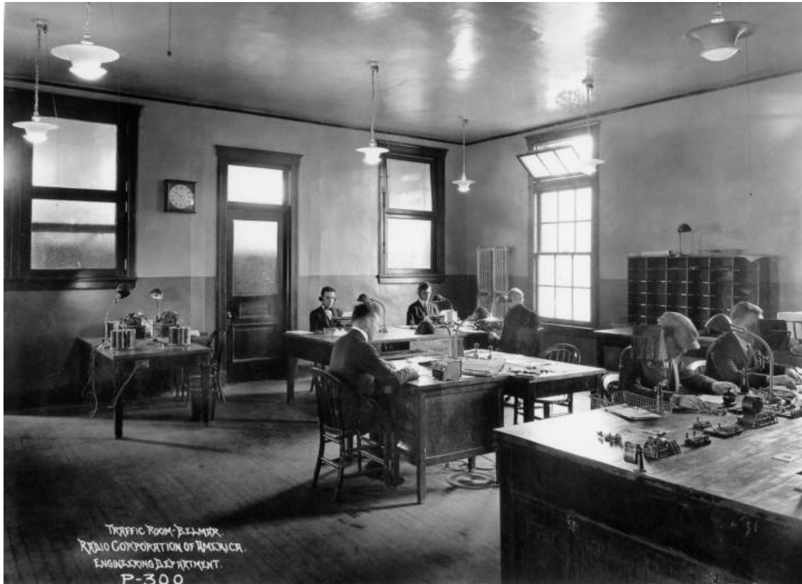
Belmar Operations Building pictures.
